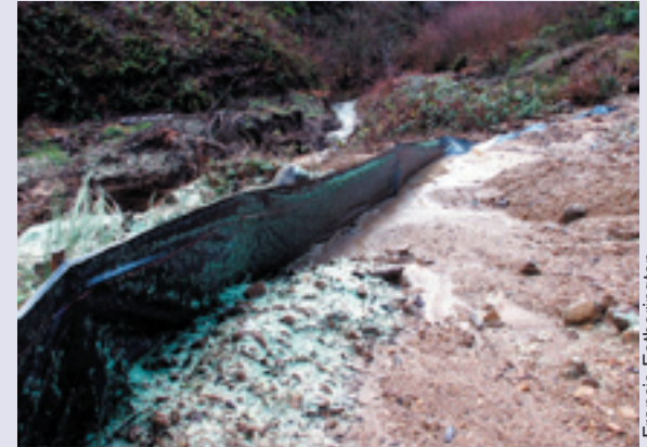
SOMETIMES MITIGATION ISN'T GOOD ENOUGH: This mitigative plastic barrier was overwhelmed by sediment from the construction of the 12-inch Coos Bay pipeline in 2007. The proposed LNG pipeline is 36 inches and 235 miles long, crossings hundreds of salmon-bearing streams.
